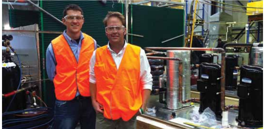
Conrad Blom (left) & Chris Elliot (right) from Selected Energy at Accent Air, Liverpool, NSW inspecting some of the units destined for the Sun City project.
